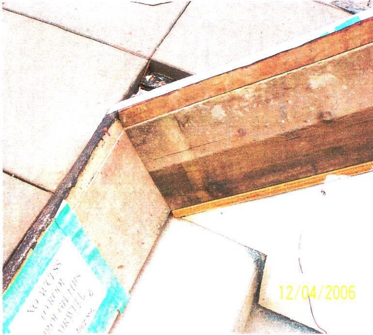
#3- Close-up of rough opening at sill/jamb area.
