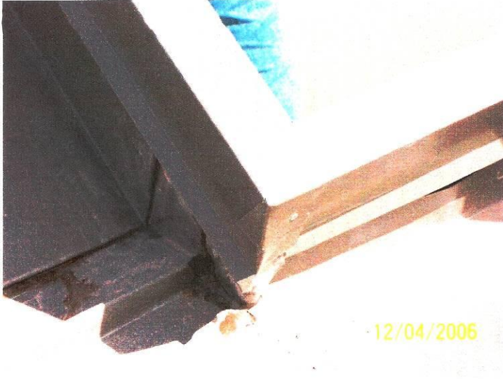
#9- Close-up view of finished jamb/sill area flashing overlap details.
