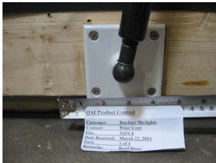
Fig. 12 – Actuator fastened to curb
